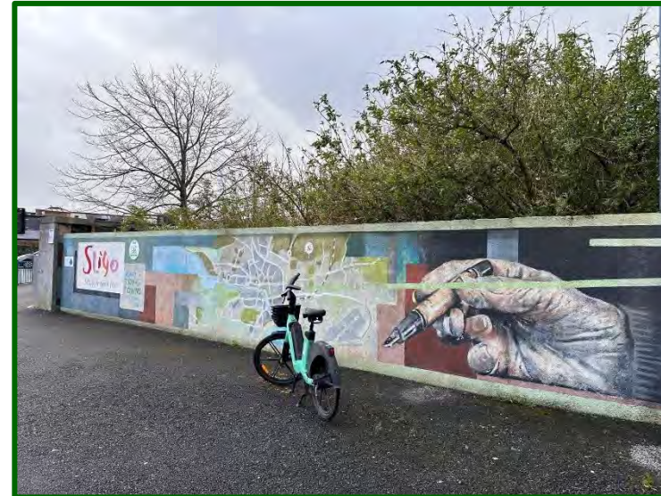
Picture 4: Stone Walls and Other Stonework (BL1) at northern boundary of the site
